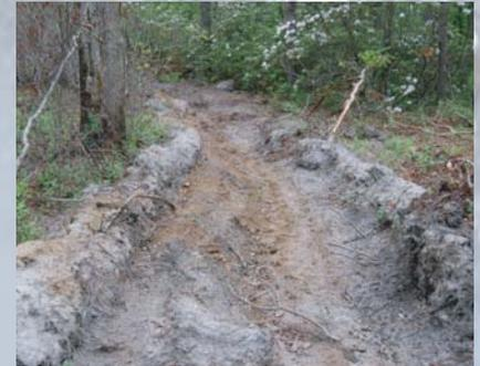
Fireline construction is most often done by bulldozer with an attached plow. In rocky areas fireline construction may be done by hand.
